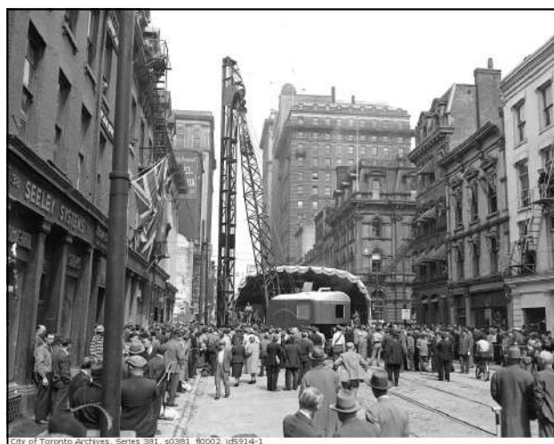
Ground breaking for Yonge Subway construction, 8 Sept 1949. Yonge & Wellington Streets. CTA
